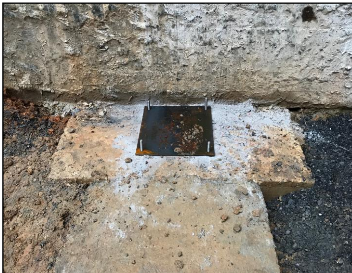
Setting Anchor Bolts
