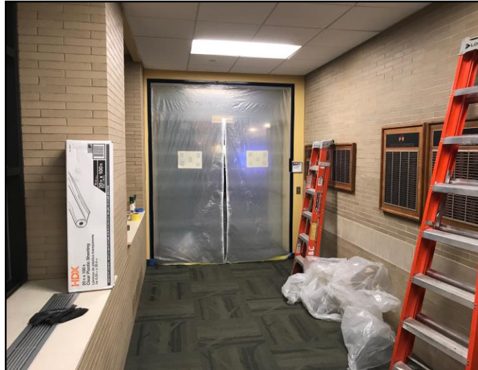
Temp Barriers Being Installed at Pattee
