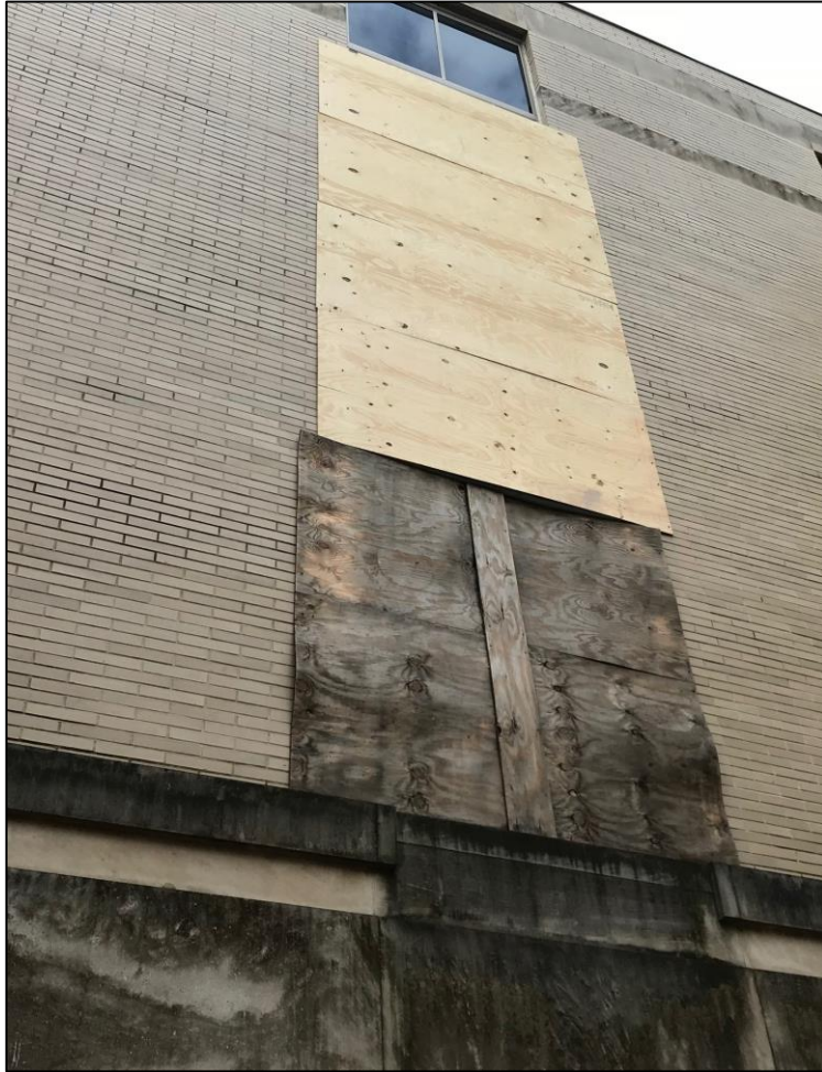
Temporary Window Protection at Courtyard
