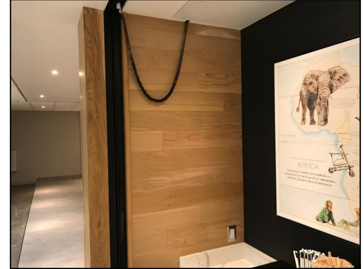
Paint Near Grille at Condiment Counter
