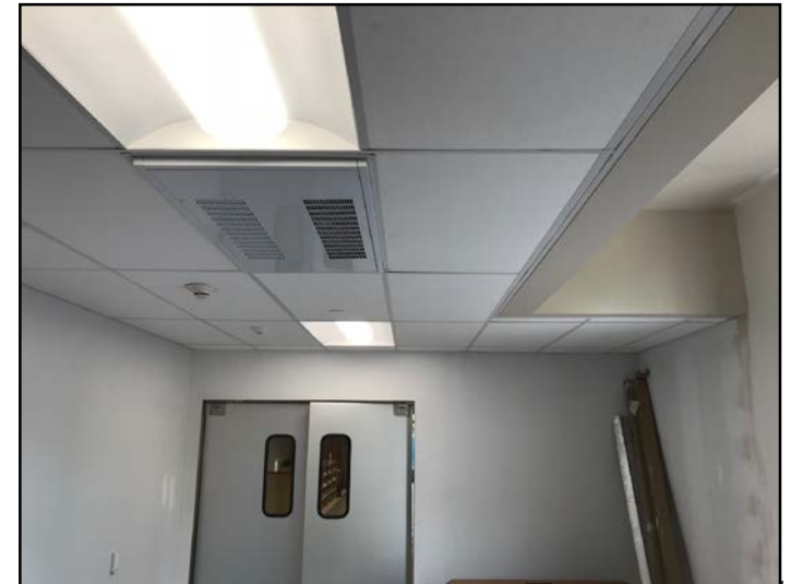
Trash / Recycle Room Ceiling Tile Complete
