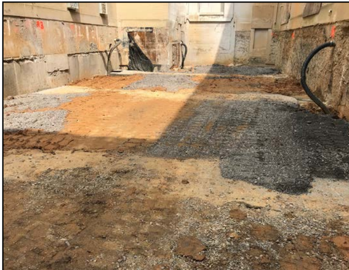
Grade Beams Backfilled
