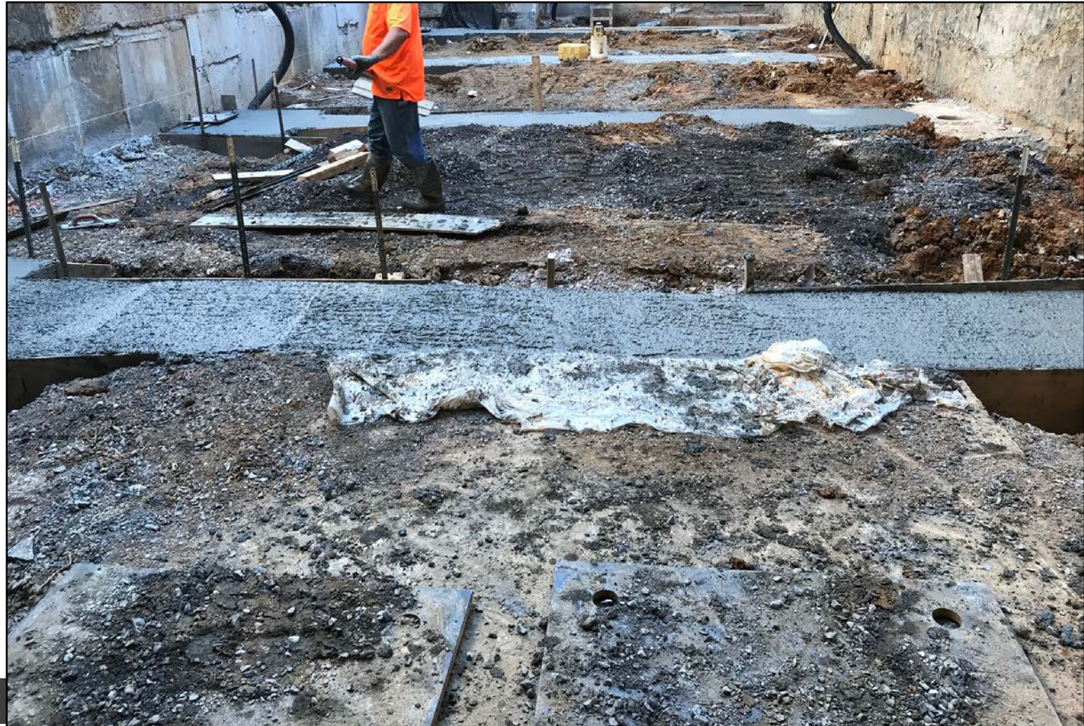
GRADE BEAM FOUNDATIONS COMPLETED
