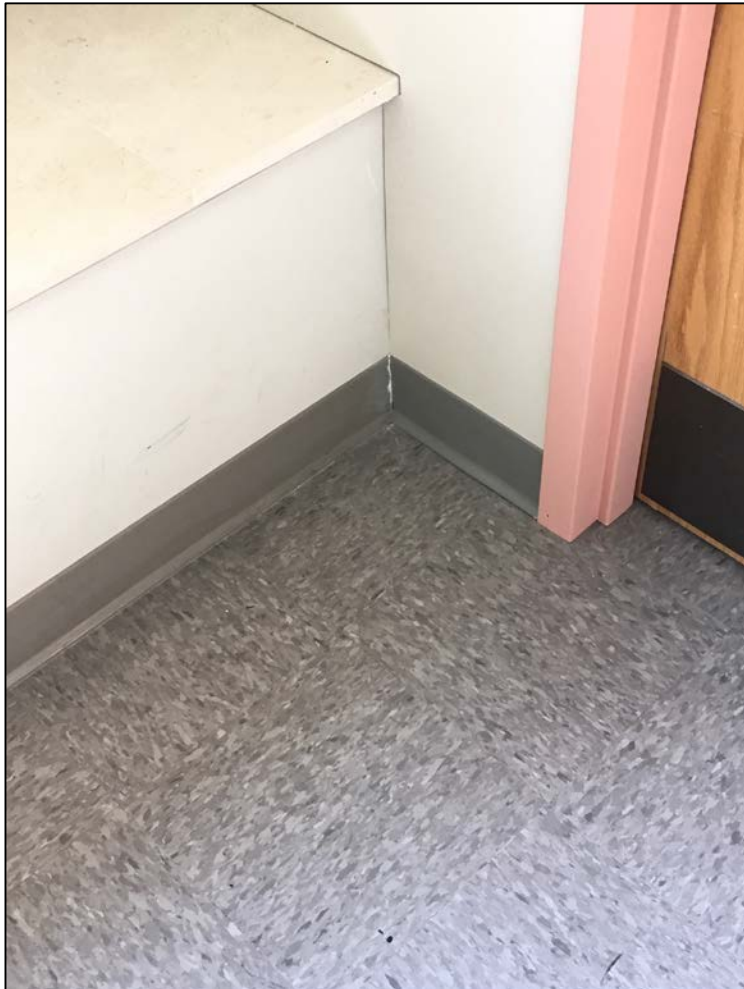
Wall Base Installed at Special Collections Door
