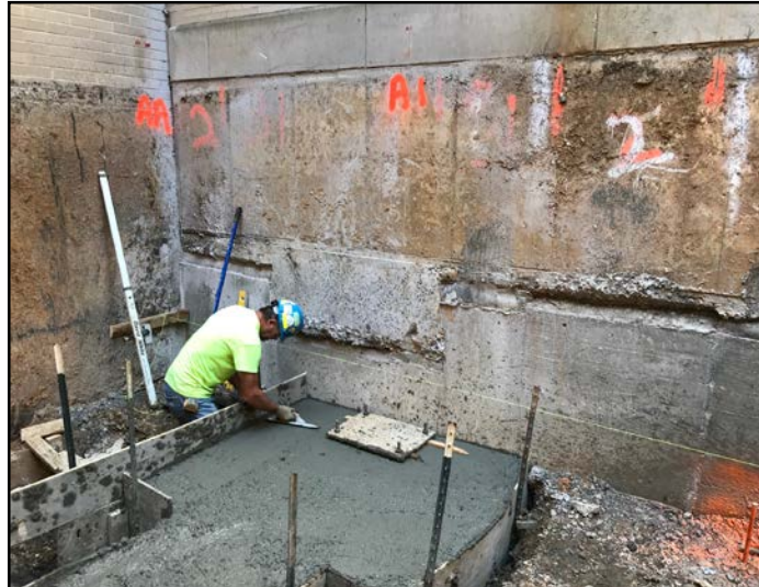
Finishing Grade Beam Concrete
