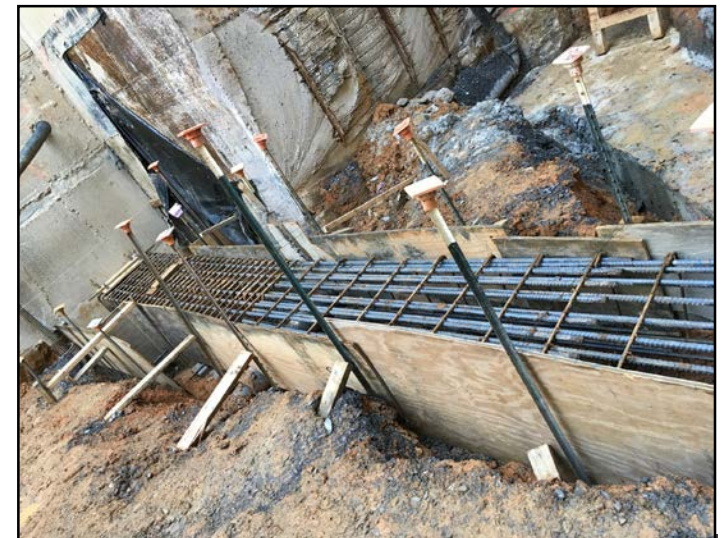
Rebar and Formwork for Grade Beams
