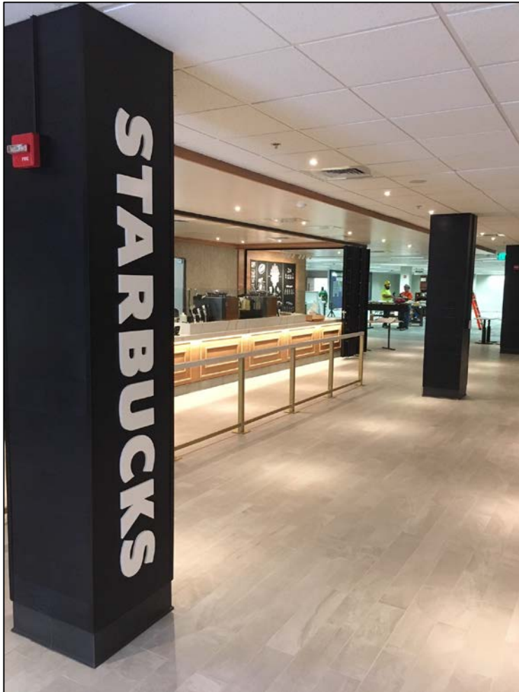
Starbucks Sign and Que Rail Installation
