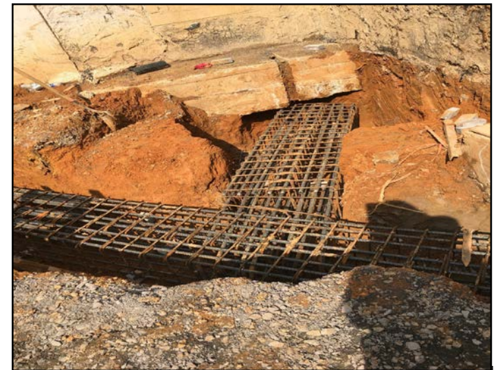
Rebar Placed for Grade Beam Foundations
