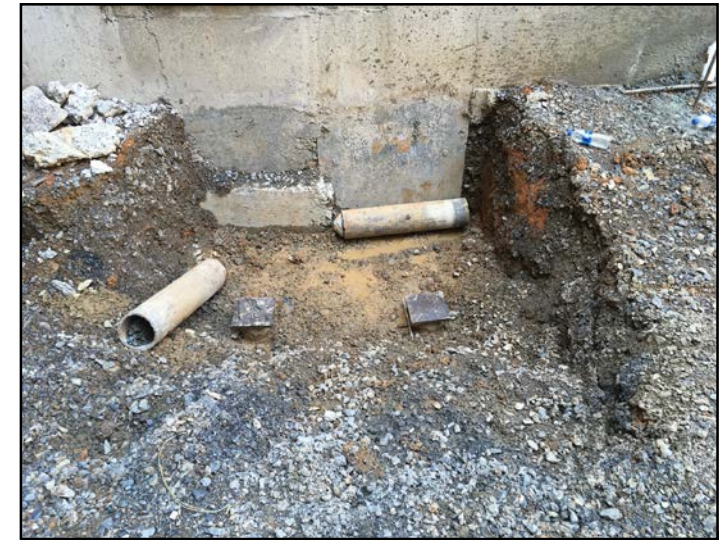
Micropiles Cut and Capped
