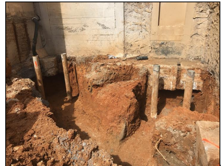
Excavation for Grade Beam Foundations
