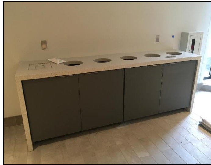
Trash & Recycling Casework Installed
