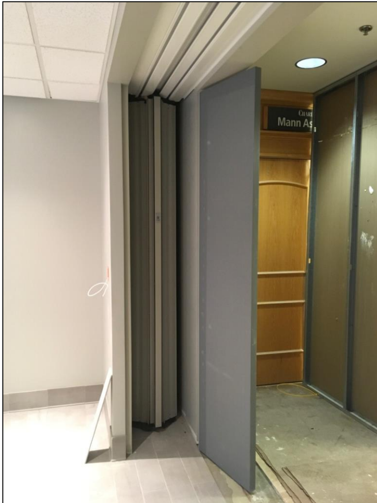
Won Door Installation Complete
