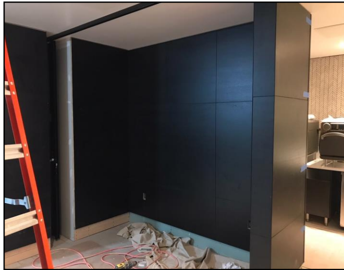
Wall Paneling Install at Reach-In Coolers
