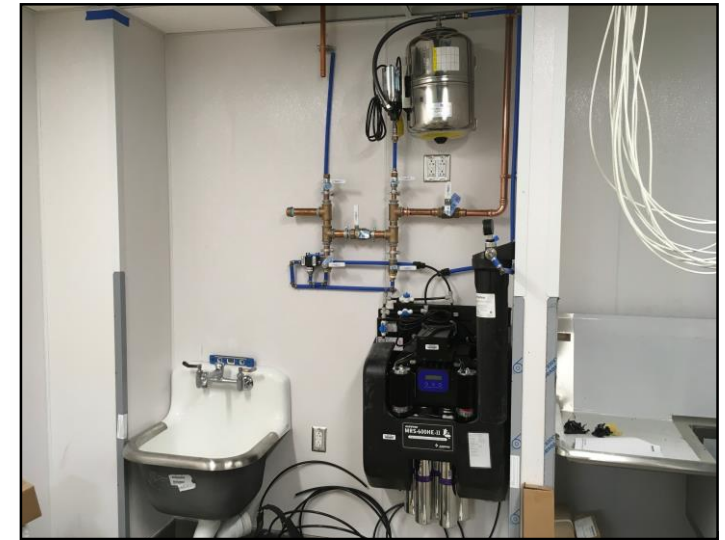
Water Filtering System Installation
