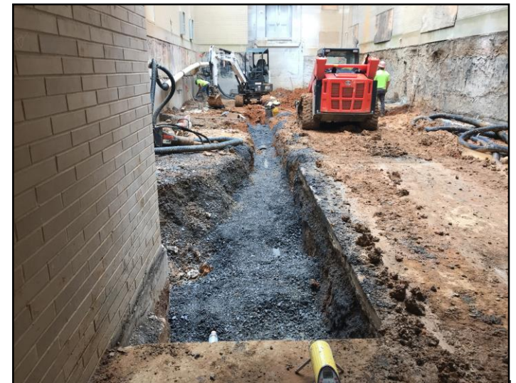
Storm Pipe Tie-Ins at Courtyard Ongoing
