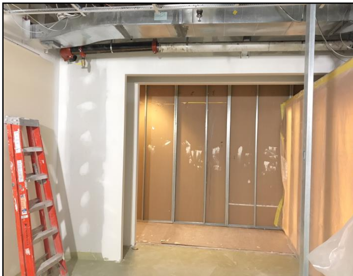
Framing at Won Door Area Complete
