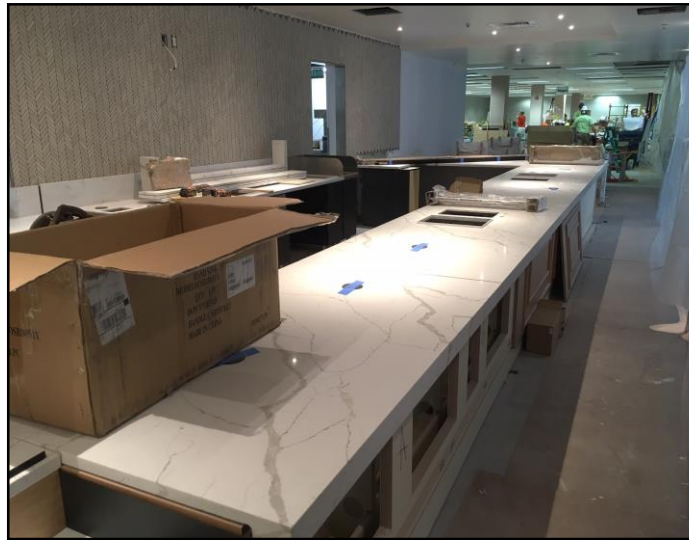
Starbucks Casework Install Ongoing
