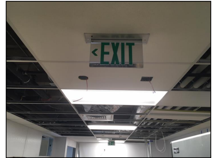
Exit Lights & Lighting Fixture Installation
