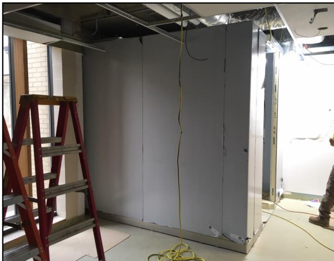
Cooler / Freezer Install Ongoing
