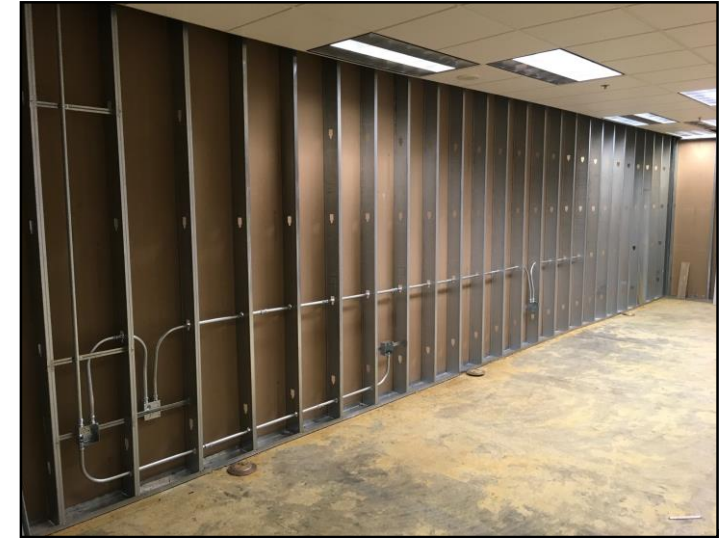
Beginning Rough-Ins at First Floor Paterno
