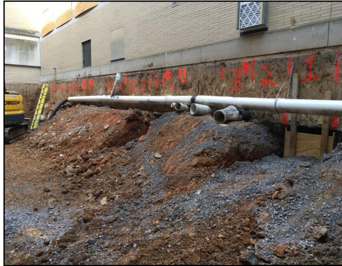
Underpinning Layout & Formwork
