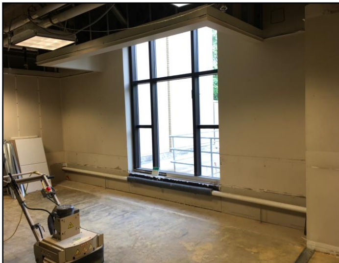
Demolition at New Storefront Area
