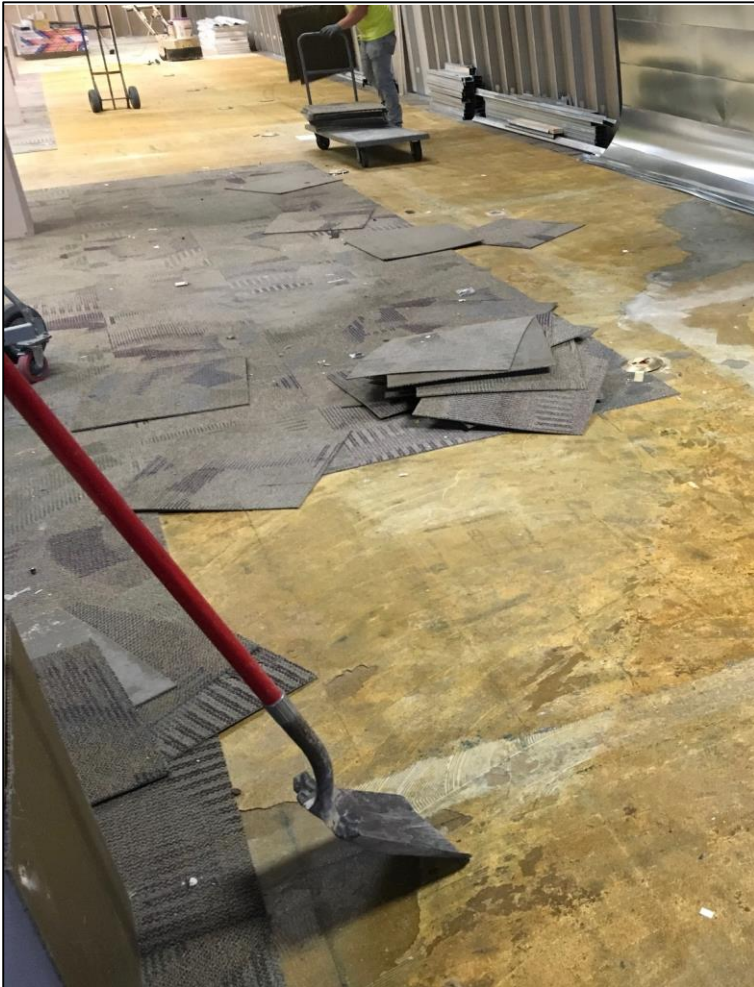
Existing Flooring Demolition Complete
