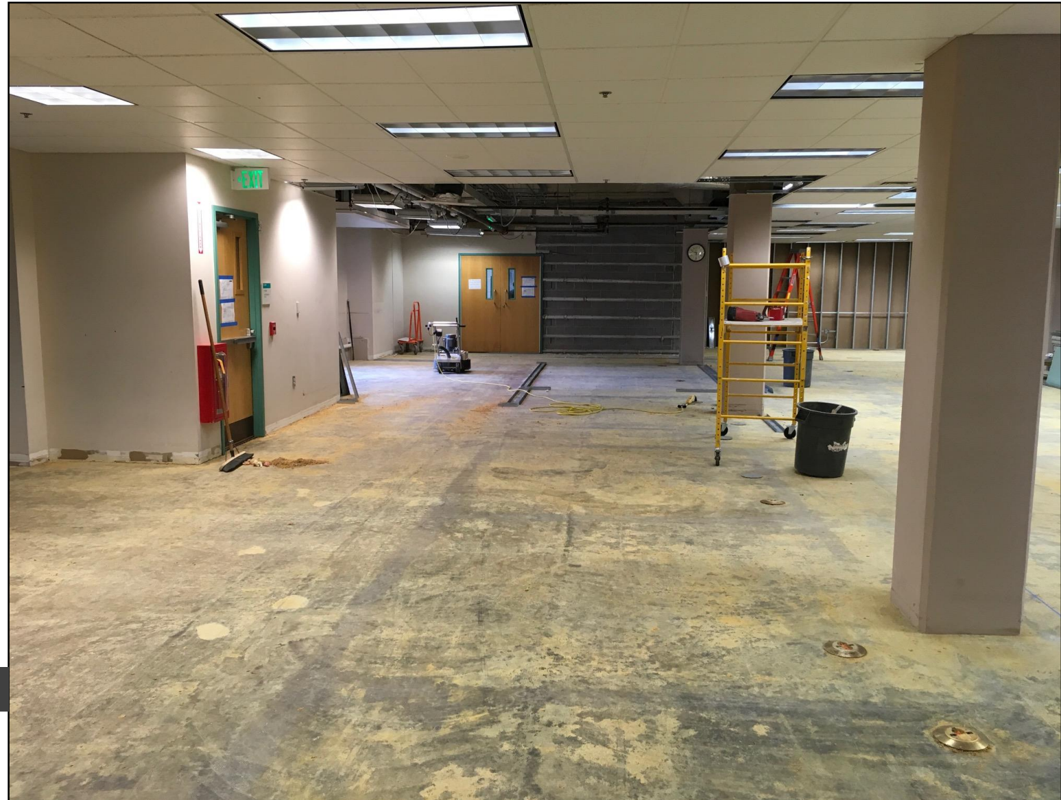
FIRST FLOOR PATERNO DEMOLITION
