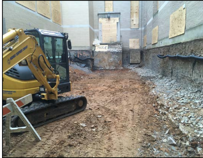
Continuing Excavation at Courtyard
