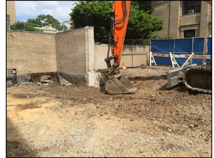
Demolition and Excavation at Terrace Stairs
