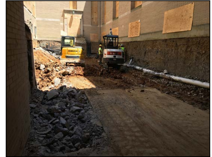
Excavation Continuing in Courtyard
