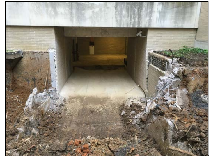
Demolition of Stairs & Walls in Courtyard
