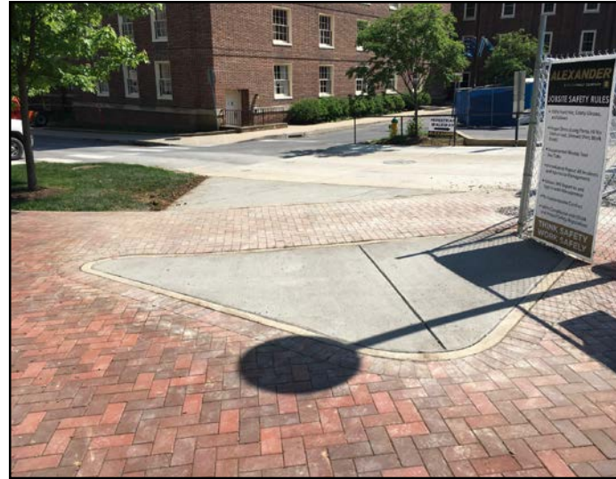
Temp Sidewalk Infills at Fraser Gate
