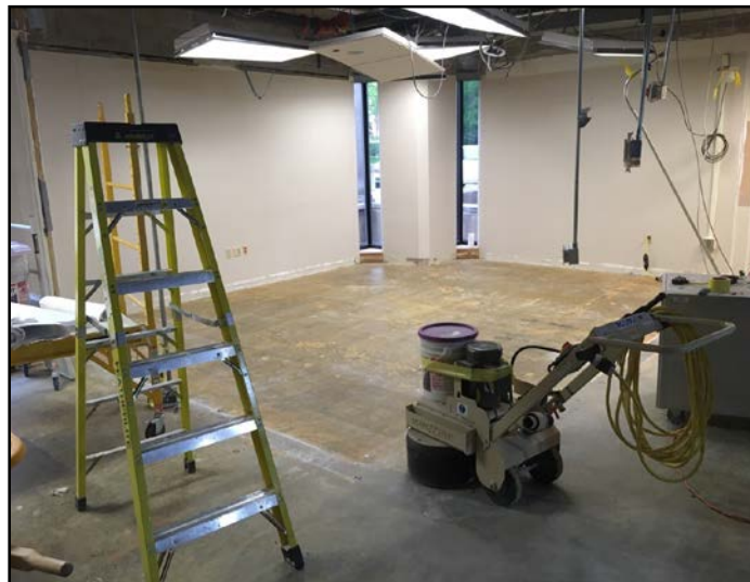
Demolition at First Floor Paterno
