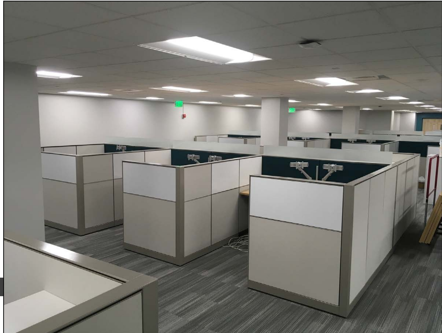
CUBICLE & FURNITURE INSTALLATION AT GROUND FLOOR
