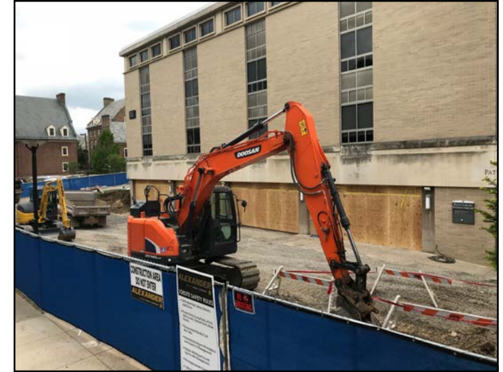
Terrace Demolition & Site Gravel Laydown
