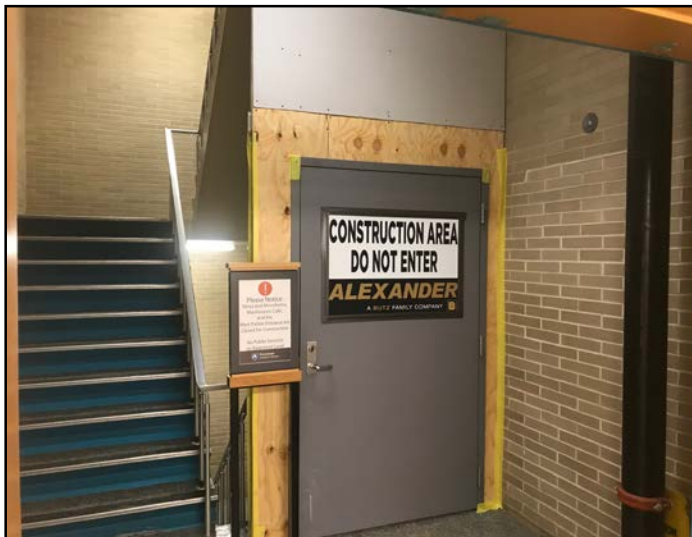
Signage & Temp Walls Erected in Pattee
